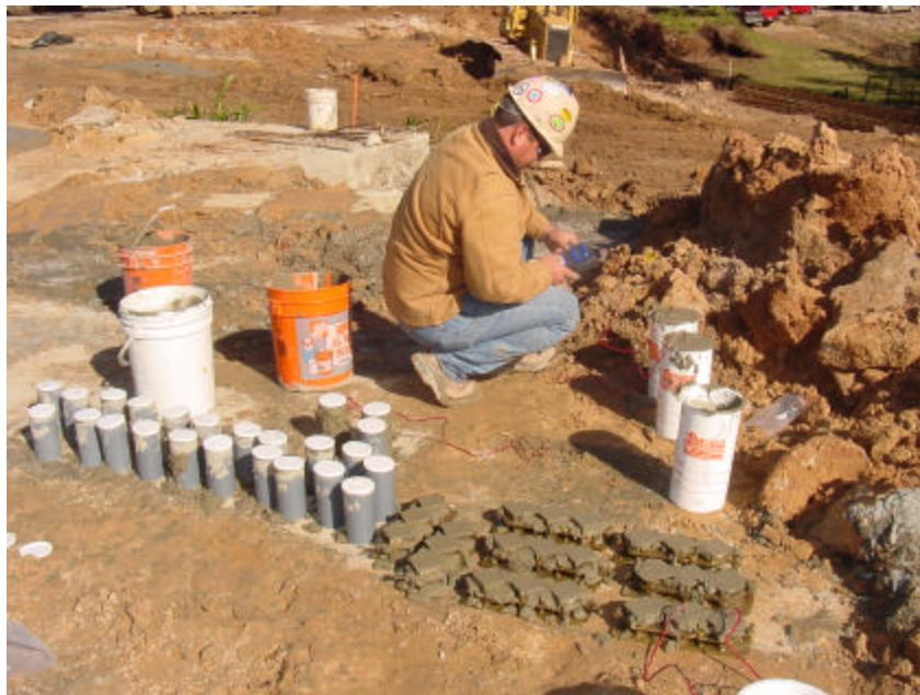
Figure 5. Collecting Grout Samples and Recording Maturity Readings
