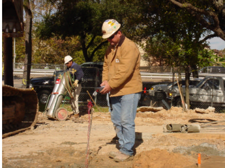
Figure 6. Maturity Readings of In-Situ Grout within ACIP Pile
