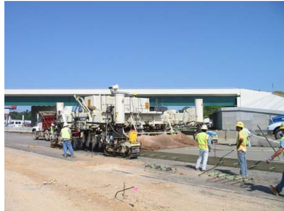
Duit crew places temporary pavement for the I-30 job.
