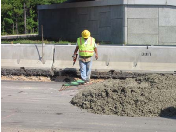
Placing temporary concrete pavement for I-30 project.
