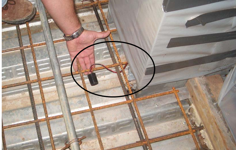
Figure 4-2 Data logger Installation Prior to Concrete Placement
