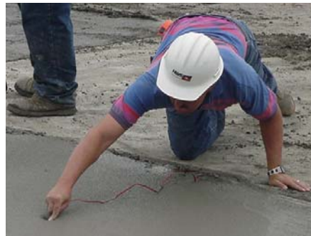
Figure 3-4: Placing an IntelliRock maturity logger into pavement
