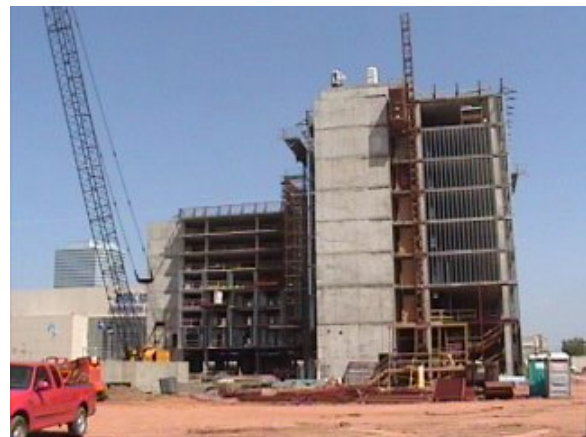
Job site in downtown Oklahoma City, April 2003.
