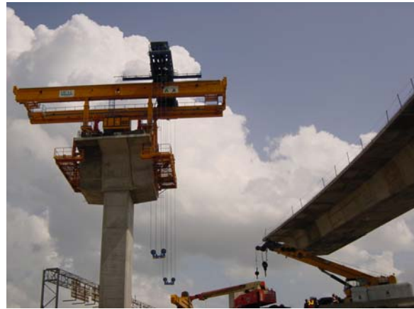
Dallas High Five Construction Site.
